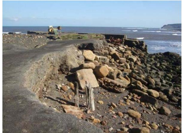
Outflanking and erosion occurring behind the breakwater
