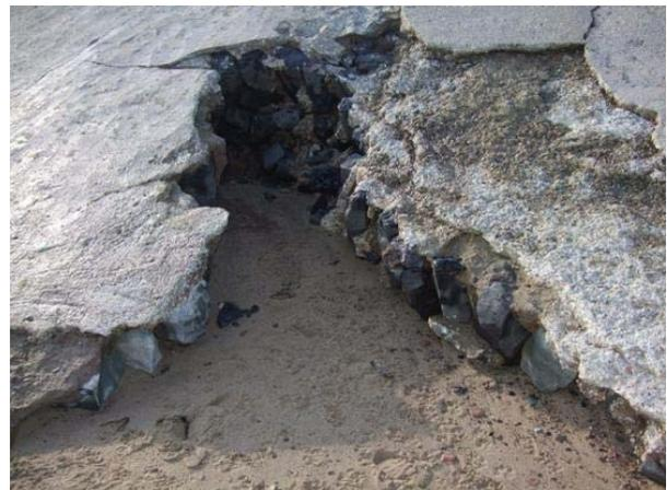
Undercutting and erosion of the concrete revetment backing Sandsend Beach (Asset Ref No. 1221D901D0702C04)
