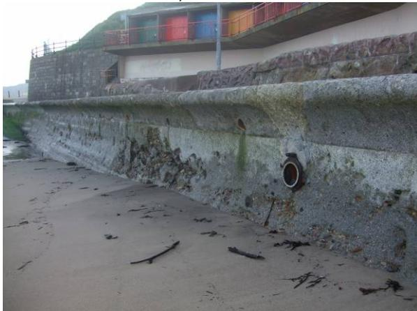
Lower section of concrete wall with significant surface erosion
