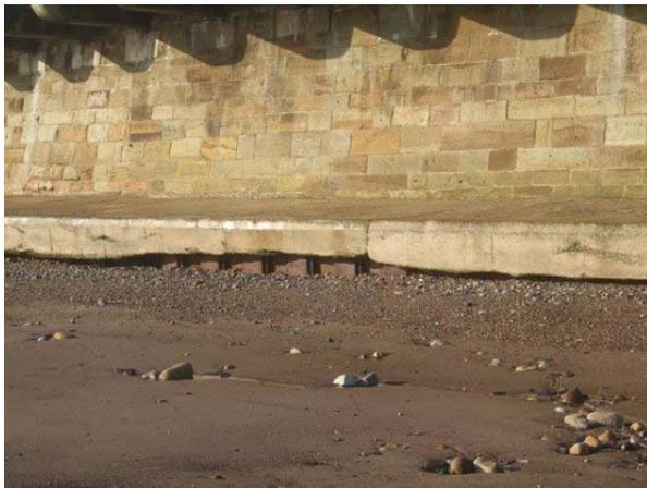
Relatively new blockwork sea wall with undercutting at the toe (Asset Ref No. 1221D901D0702C04)
